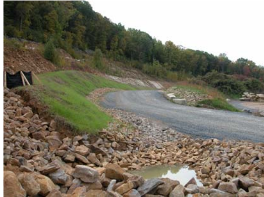
Quarry roads are laid with gravel to minimize dust, and scrap stone is used to create drainage ditches as well as provide support to the adjacent hillslope.
