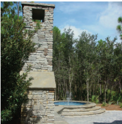
Flagstone Slab Roofing
